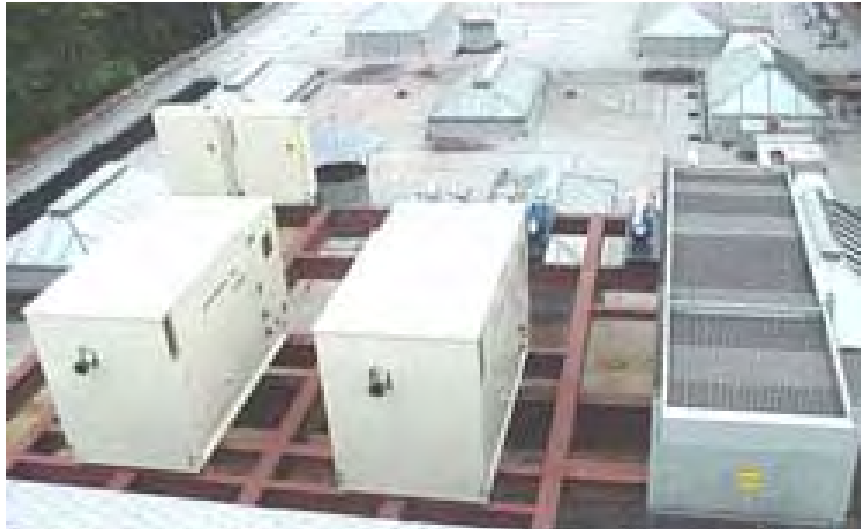
Mechanical Platform. 2-150 kW Generators and Fluid cooler
